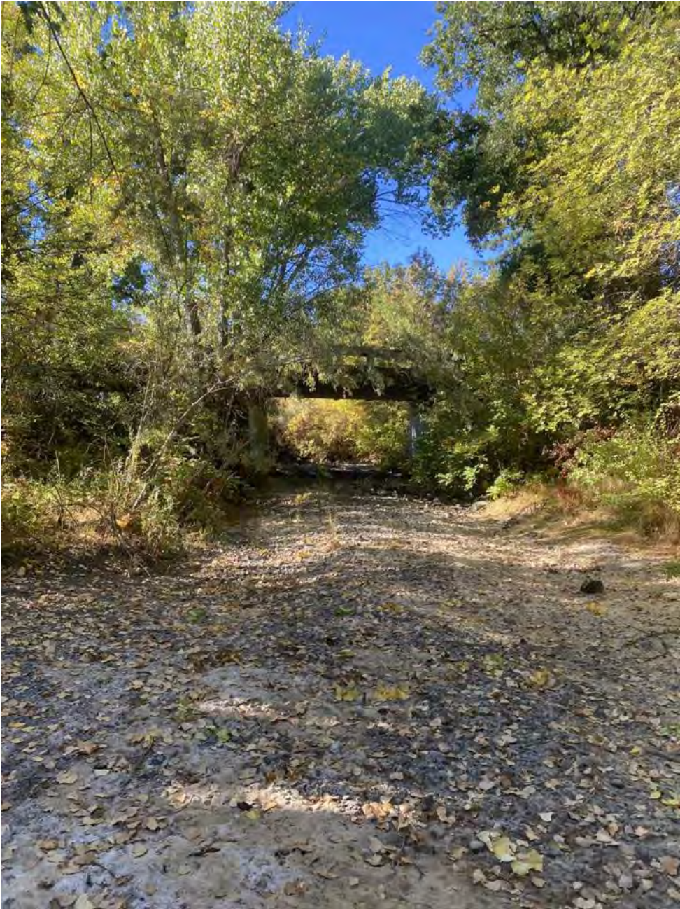
SITE 1- LOOKING DOWNSTREAM.
